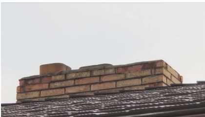
Cracked bricks
